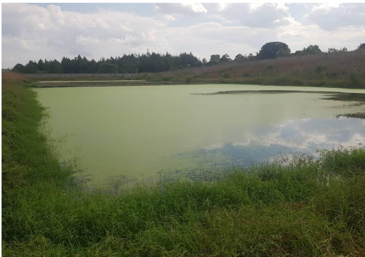
Figure 5.17: Wastewater Stabilisation Pond at Mzuzu University
