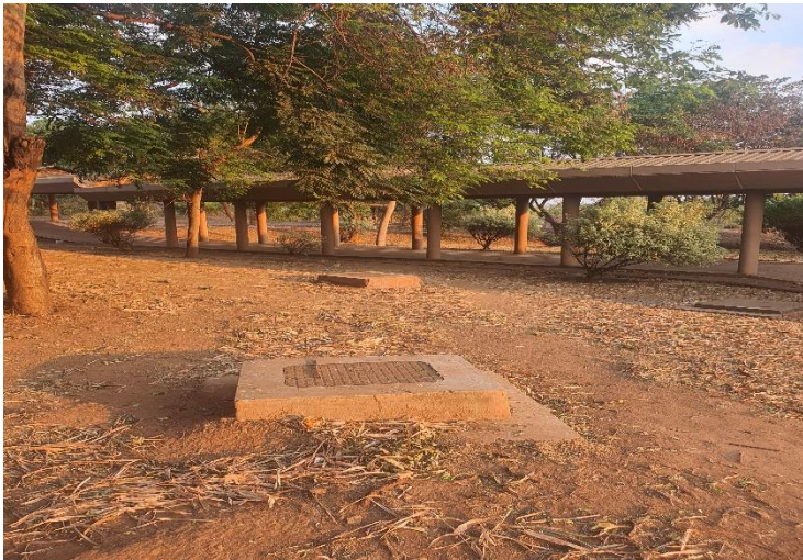
Figure 2: Manholes leading to main public Sewer line likely passing through the project site
